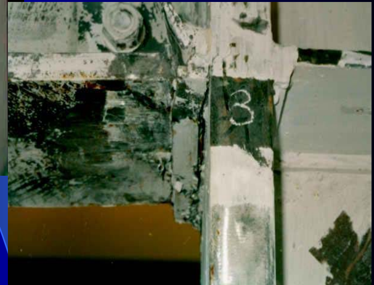
Brittle damage through base metal of the column flange and panel zone
