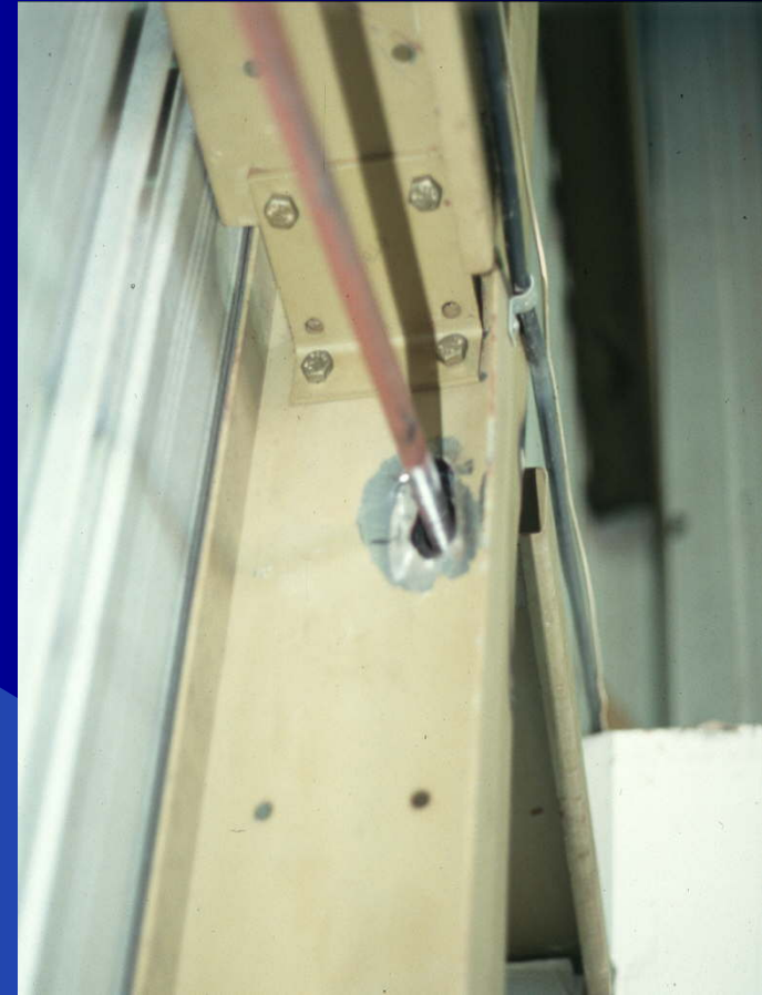
Hole Ovalization of slender bracings formed from rods (Northridge, 1994)
