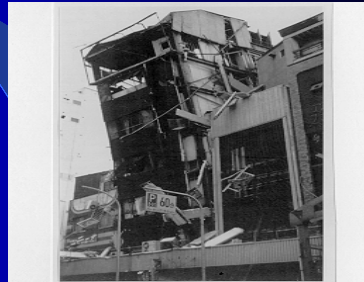
Fig. 6.91 Excessive sway due to fracture of slender braces
