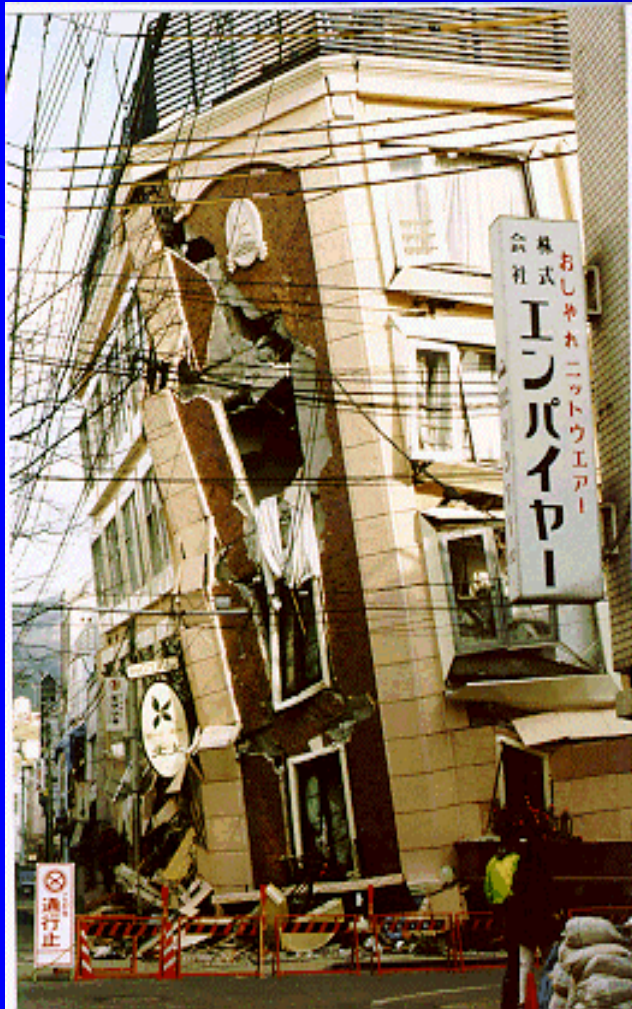
Tily up of a steel building (Kobe Earthquake, 1995)
