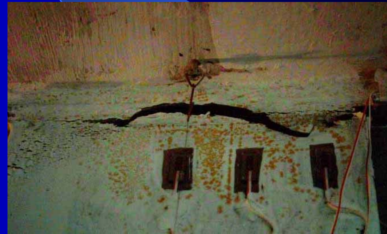
Brittle damage through base metal of the column flange
